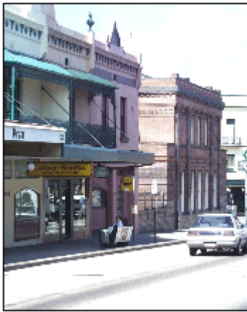
Retain face brick details of important buildings such as the former National Australia Bank and original balconies
