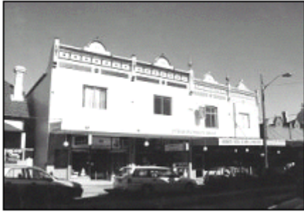
Federation and Inter-war buildings contribute to the centre's character.
