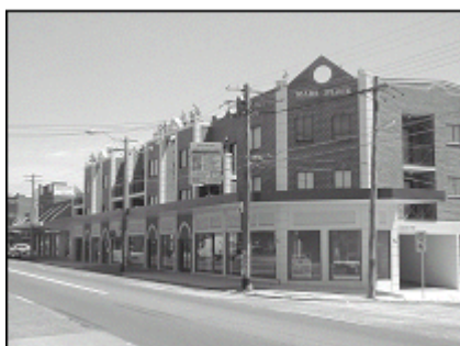
New Canterbury Road, Hurlstone Park
