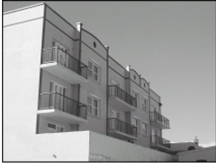
Open space areas such as balconies are to be orientated to the north for maximum solar access
