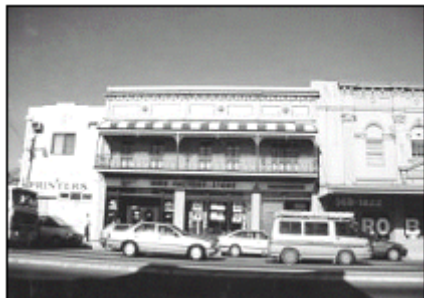
A successful example of a verandah restoration, has significantly improved the visual presentation along this part of Parramatta Road.
