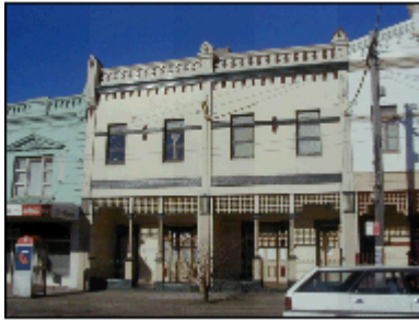
Example of traditional parapets creating a repetitive pattern and interesting skyline.
