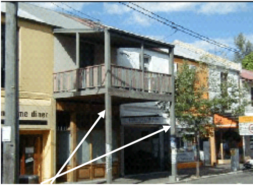
All structures shall be designed to be self supported in the event of removal of the post(s).
