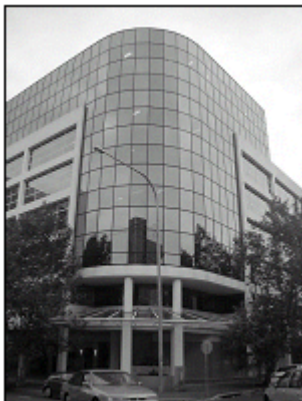
NOT RECOMMENDED: X Large expanses of glass curtain walls and reflective wall cladding
