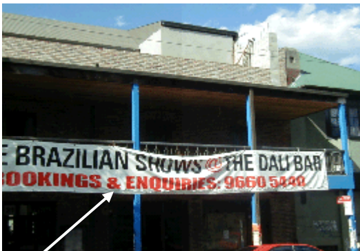
NOT THIS Signage which obscures the architectural features of the structure and building.
